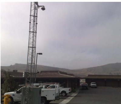
Outdoor IVC PTZ camera and wireless radio mounted on tower to monitor building and facility access and parking lot.
