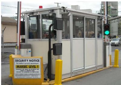
"Cost and time for installation was significantly reduced using IP cameras. This enabled use of power over Ethernet for indoor cameras and wireless LANs for the cameras that reduced need for cabling and trenching."
